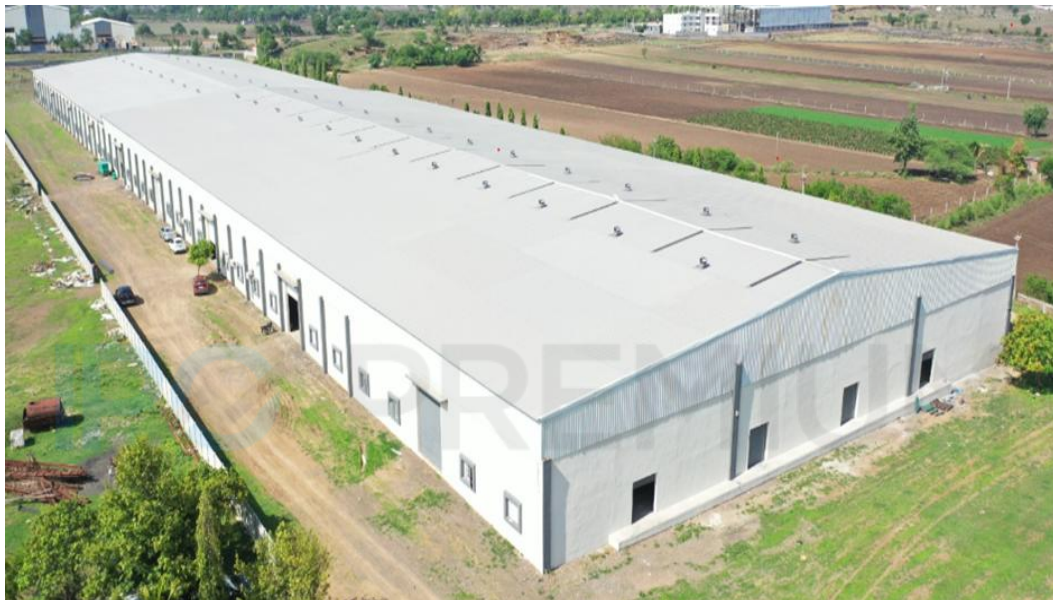
(Padavala / Existing Facility 3)
